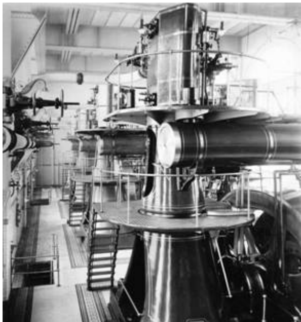
Bristol Tramways Power Station Dynamos 1900
